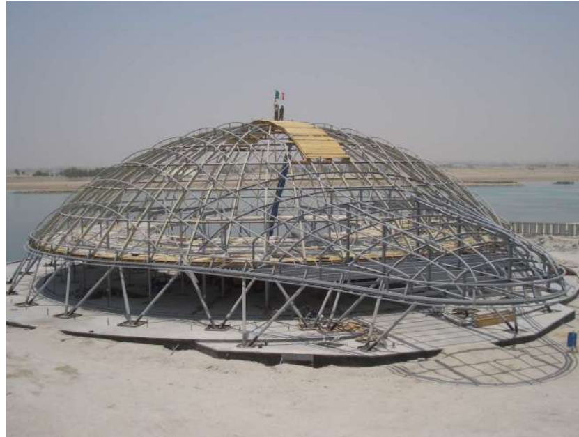
THE PEARL QUATAR. On site erection phase
