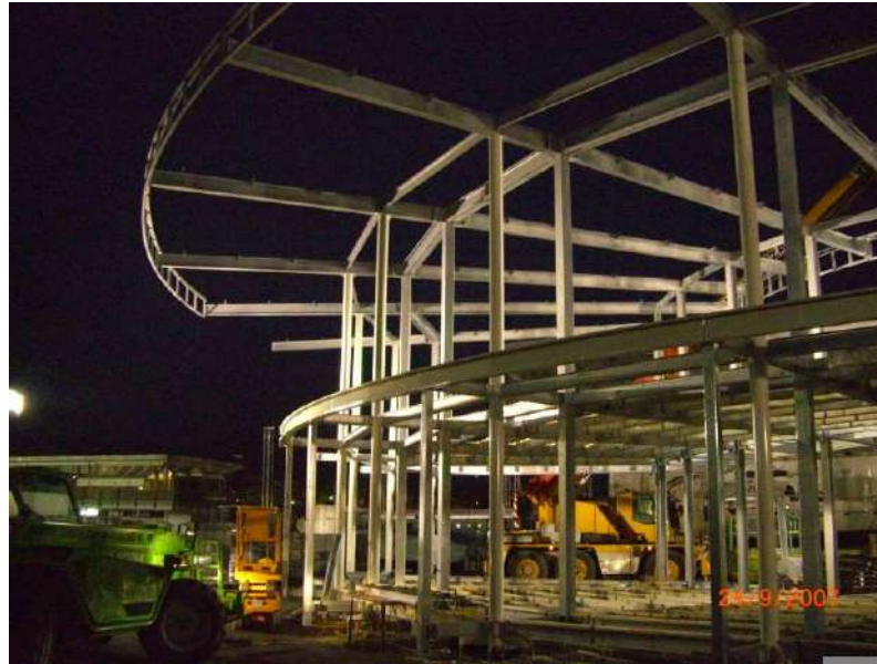
STAND FERRETTI NAUTICAL EXHIBITION GENOA. On site structural steelwork erection phase
