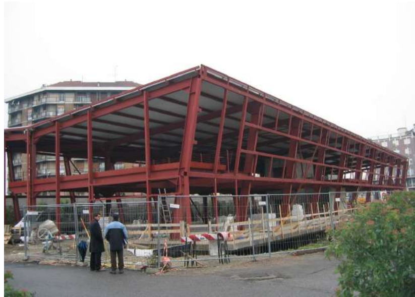
SHOW-ROOM FASSINA MILAN On site structural steelwork erection phase
