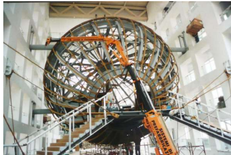
EXPO SIVIGLIA 1992 On site structural steelwork erection phase
